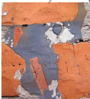
A special flexible polymer filling cracks of a damaged masonry
